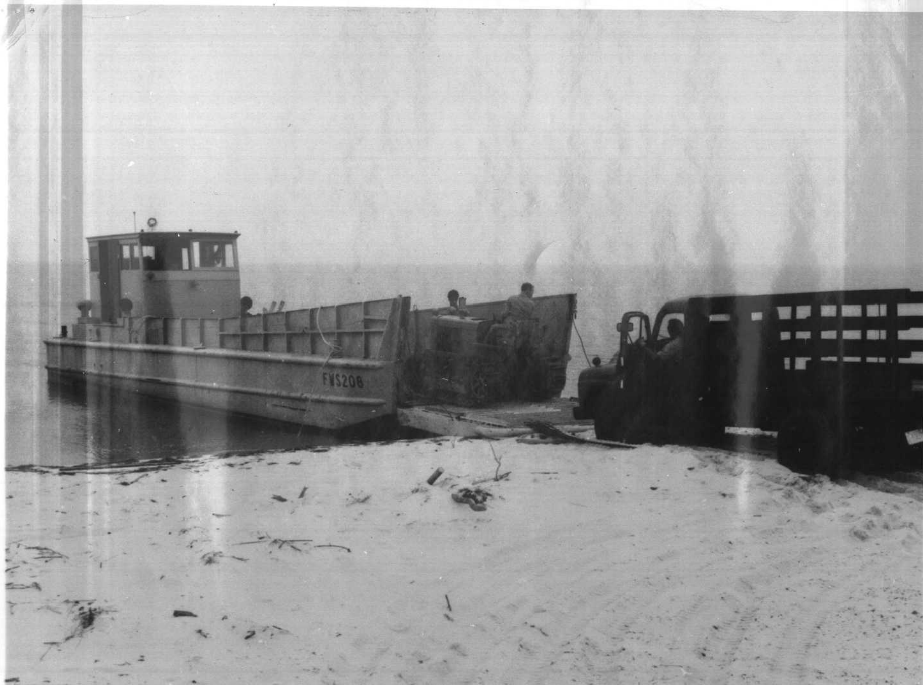
An LCM is used to haul equipment and supplies from the mainland to the islands. Although slow, it is ideally suited for operation in the shallow waters adjacent to the islands. Movement of personnel, supplies and equipment on the islands themselves constitutes a problem in the soft sand. Crawler tractors have to be used to assist regular highway equipment from point to point. Shifting sand on the beaches make it impossible to provide a hard surfaced roadway.
