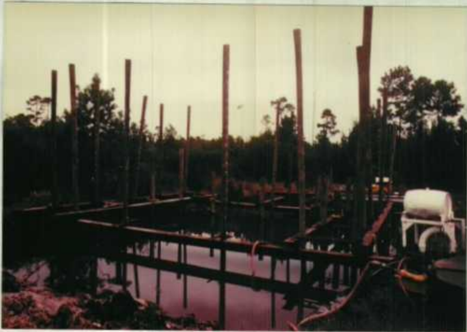
New boathouse construction at Kingfisher Landing - October, 1979. (TW) 8-OKE-79
