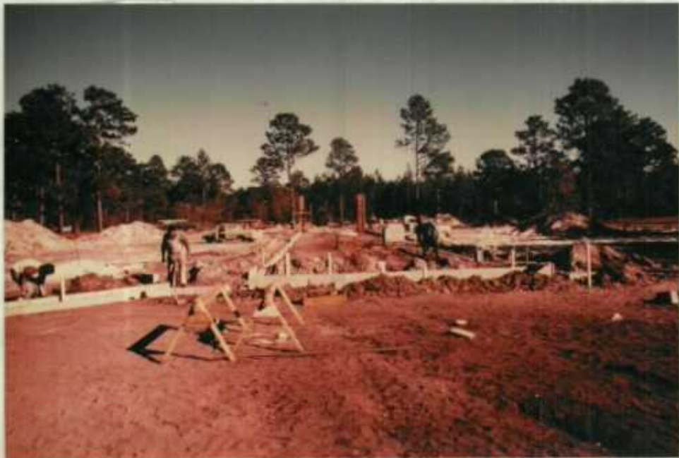
Construction work begins on new headquarters at Camp Cornelia - December, 1979. (TW) 9-OKE-79
