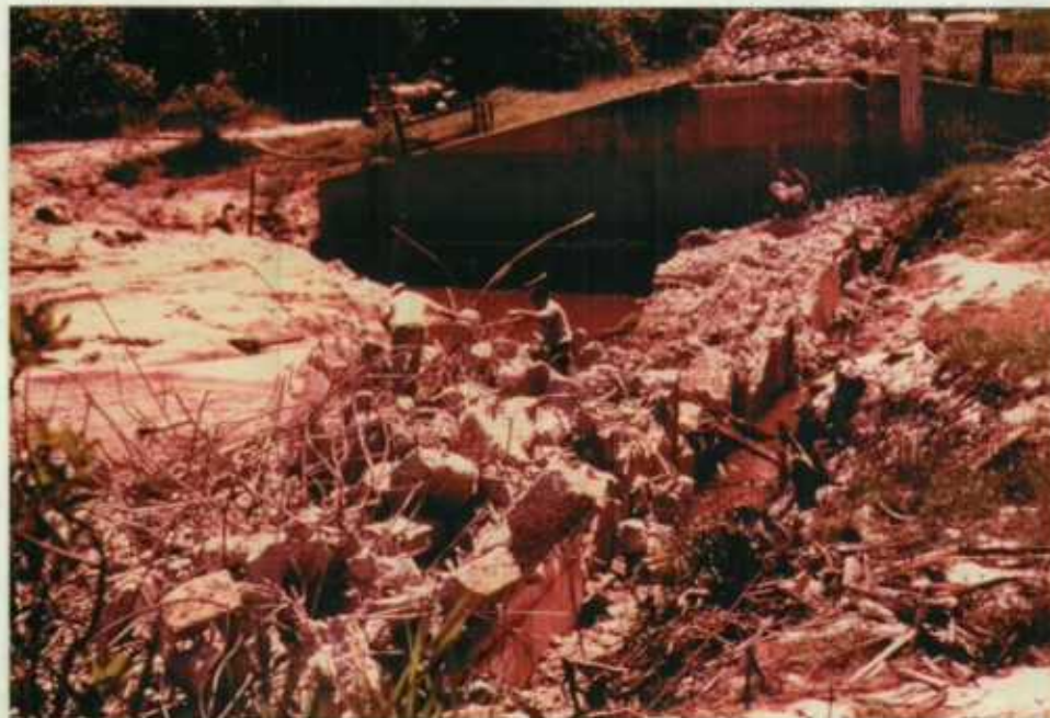
Suwannee River Sill Water Control Structure demolition and replacement. (TW) 6-OKE-79
