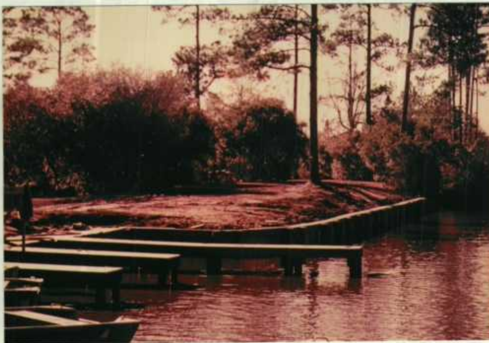
Completed bulkhead at Suwannee Canal boat basin - January, 1979. (TW) 4-OKE-79
