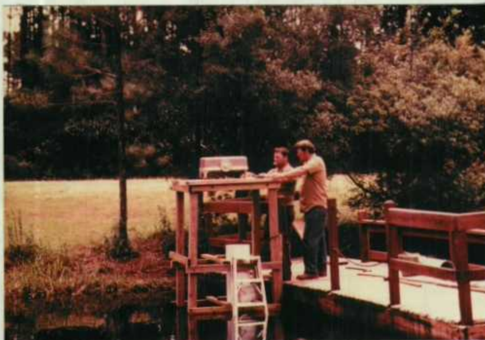
Refuge employees Phillips and Dixon installing new water level recorder at Suwannee Canal Recreation Area - September, 1979. (TW) 7-OKE-79
