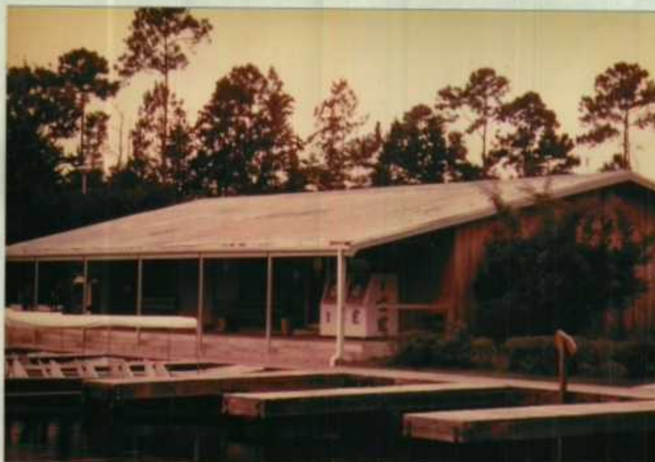
Suwannee Canal Recreation Area Concession Building prior to roofing. (TW) 10-OKE-79
