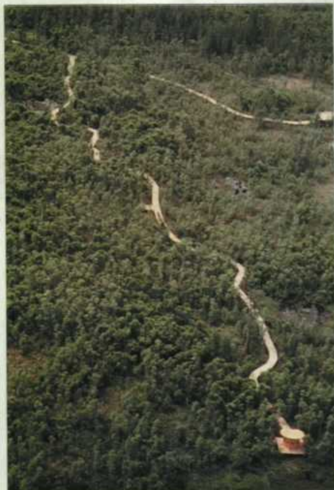
Completed Chesser Island boardwalk spur and photo- blind (foreground) (June, 1970) --(Job Order No. 2821-897-T4) (WCK) 48-OKE-79 --Right--
