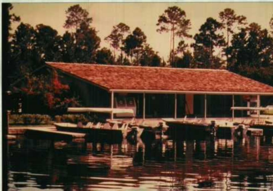
Suwannee Canal Recreation Area Concession Building with refurbished Cedar Shake roof - October, 1979. (TW) 11-OKE-79
