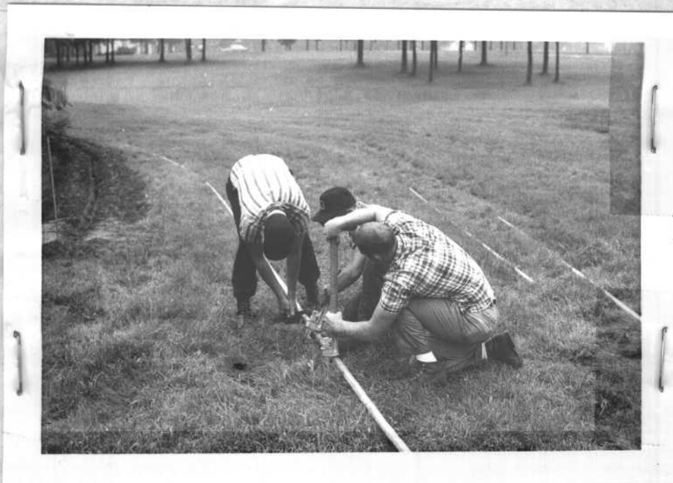
PIPELINE REPLACEMENT: To clear up the headquarters water situation, both the five hundred gallon pressure tank and the main pipeline were replaced. J. L. Darden
