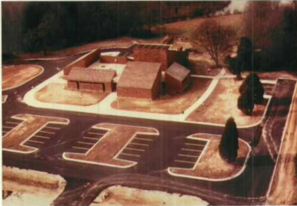
Aerial view of Wildlife Interpretive Center (WIC) nearing completion.
