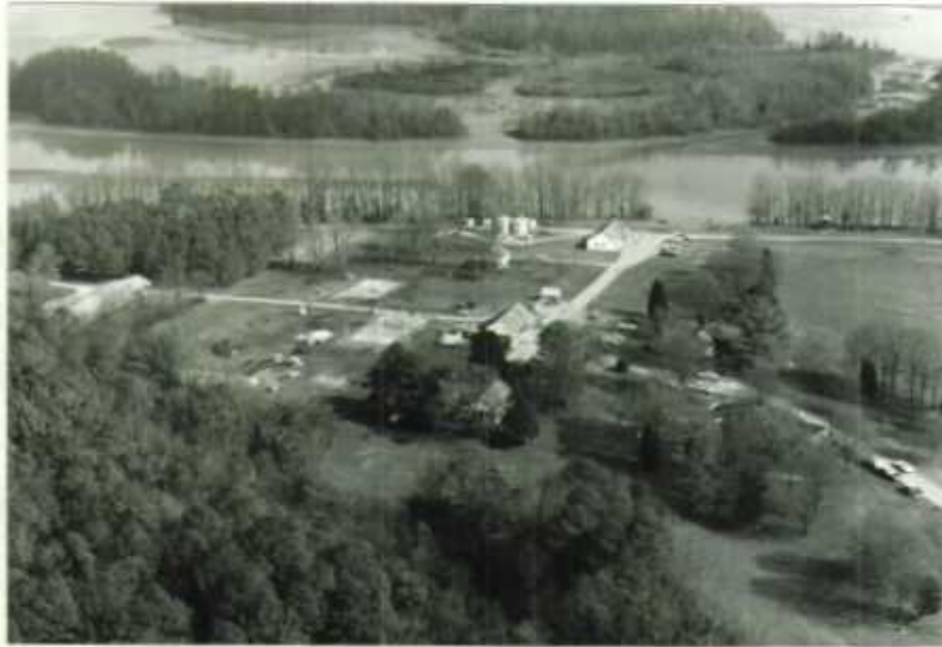
Aerial view of Headquarters showing original buildings and new buildings under construction.
