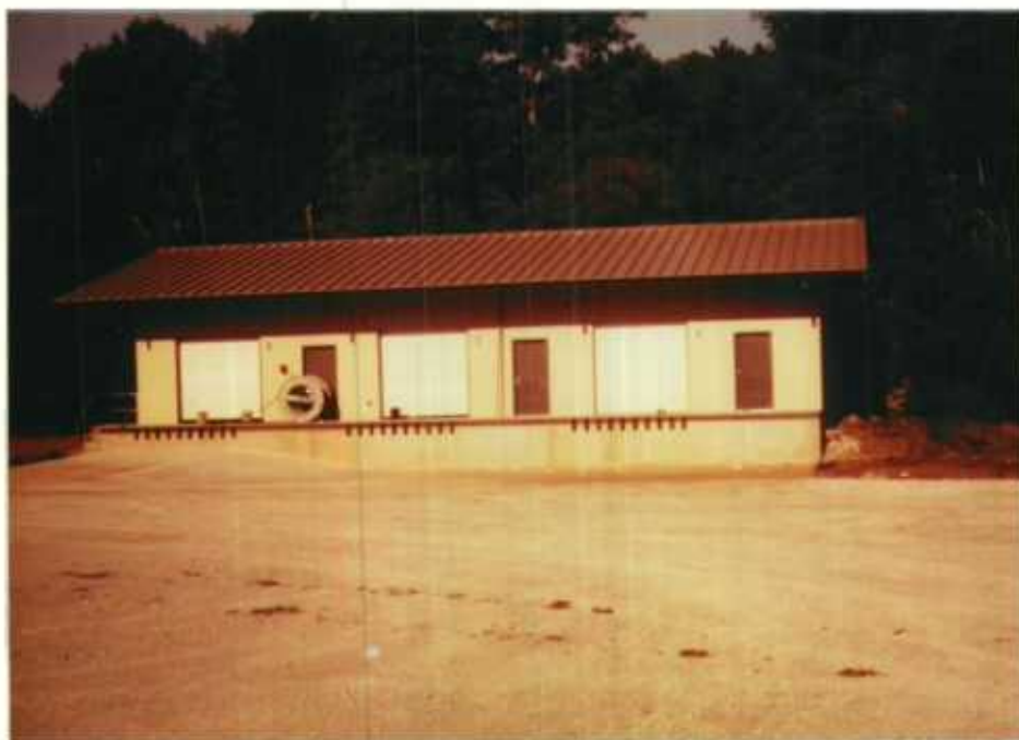
New warehouse building.
