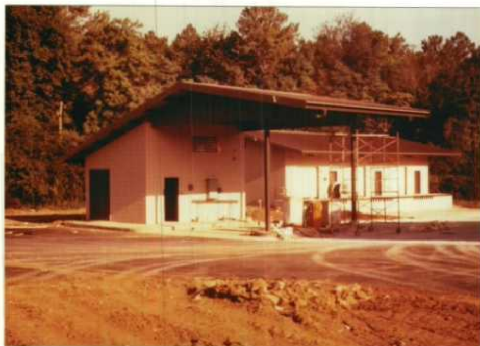
New oil house and fueling facility.
