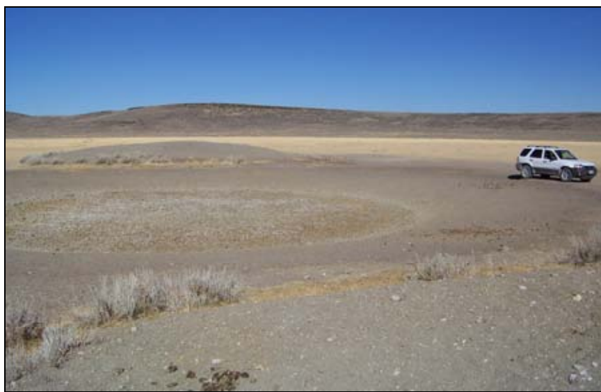
Photo 3.3 Excavated catchments or dugouts like the one shown were constructed in the middle of playas to concentrate water for livestock use (Photo Aaron Collins).
