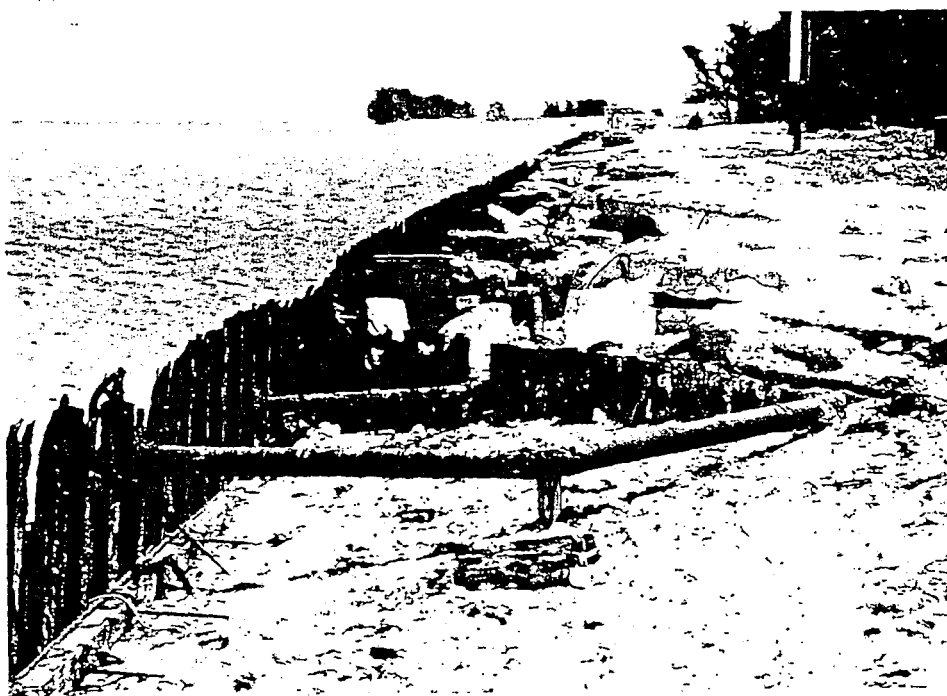
Plate III-3a. Deteriorating bulkhead, Eastern Island
