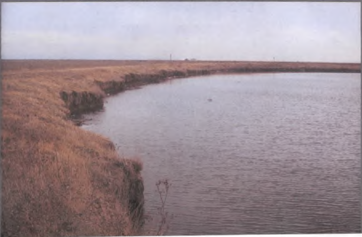
Extensive erosion and "scarp formation" along the northeast corner of the California Department of Fish & Game mitigation impoundment (below)
