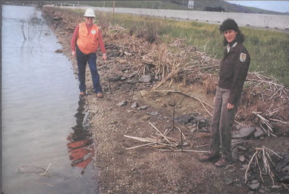
Chuck Morton, Caltrans Biologist and Louise Vicencio, Wildlife Biologist for San Pablo Bay NWR observe rebar stakes once holding several square bales of hay-- efforts to reduce erosion along the northern edge of the Tolay Creek tidal restoration project (HW 37)
