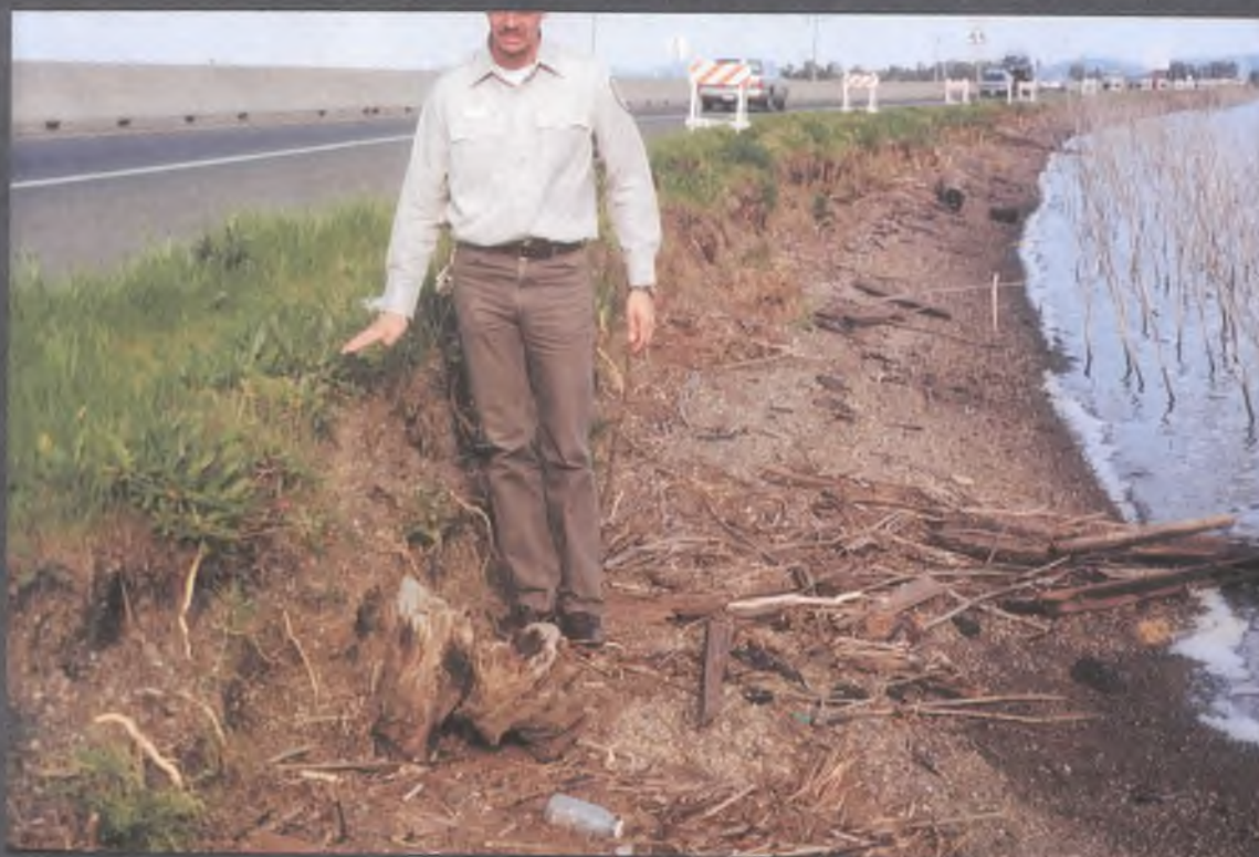
Bryan Winton, Refuge Manager, (headless) serves as reference to the areas of most extensive erosion along HW 37. The Tolay Creek tidal restoration project eroding into the roadbed of HW 37
