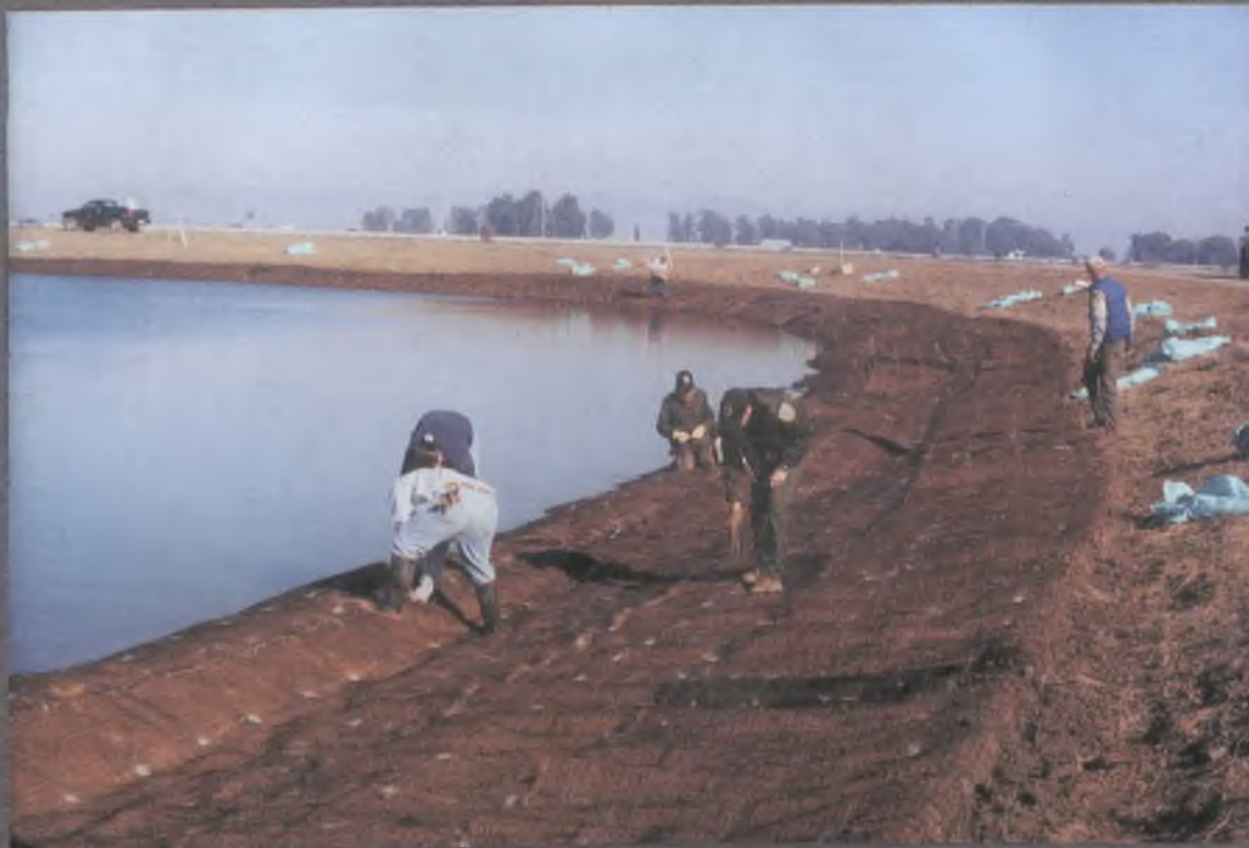
California Department of Fish & Game and Ducks Unlimited Inc. partner to install erosion-reducing fabric atop fresh fill provided by U.S. Fish & Wildlife Service (above)
