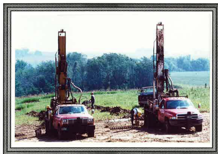
Drilling well fields for the earth-coupled heat pump at the Prairie Learning Center.
