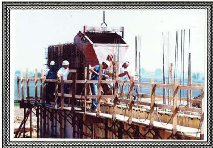
Construction workers pour the west wall of the Prairie Learning Center.
