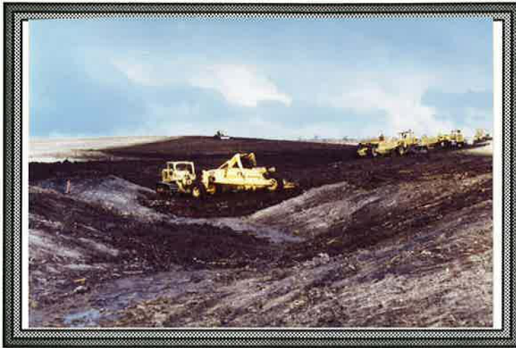
Contractor repairing gully erosion at "refrigerator gulch".
