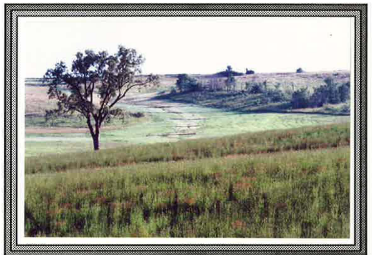
Coconut fiber matting, silt curtains, and a planting of cool season grasses stabilize the soil in a reshaped gully.
