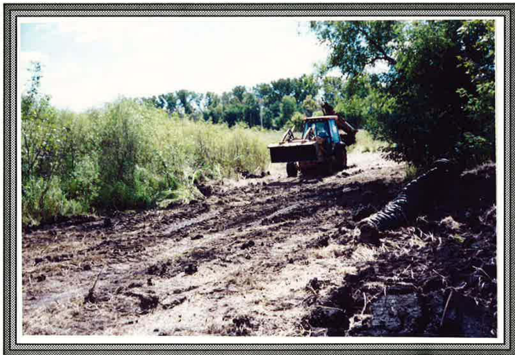
Morris Trenching & Hoe Inc. constructs a ditch plug to restore wetland hydrology on a 27 acre FmHA conservation easement restoration in Polk County.
