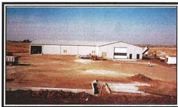
Seed and equipment storage building.
