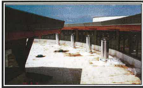
Skylights that reflect light through a tube into the bookstore. April, 1996
