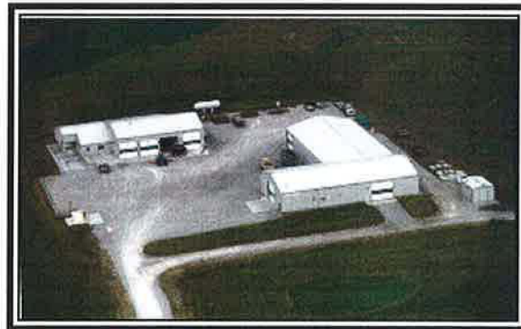
An aerial view of the Maintenance Facilities.
