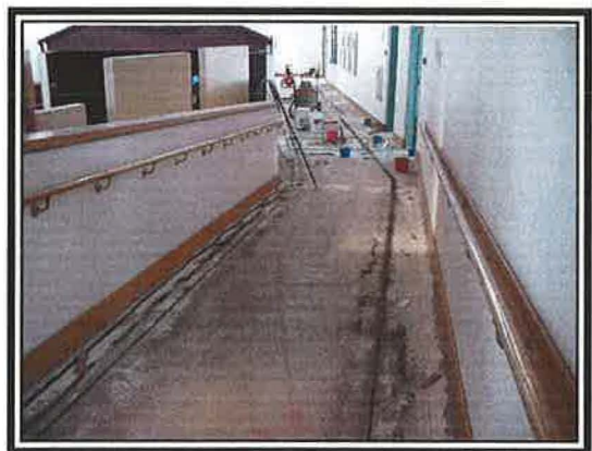
Grooves being cut into concrete floor
