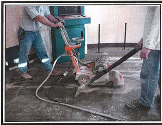
Grooves being cut into concrete floor
