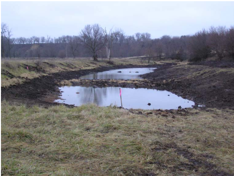
Photograph taken after completion of oxbow restoration on Cedar Creek in Greene County, Iowa. Note the gently sloping sides and relatively shallow nature of the constructed pool.
