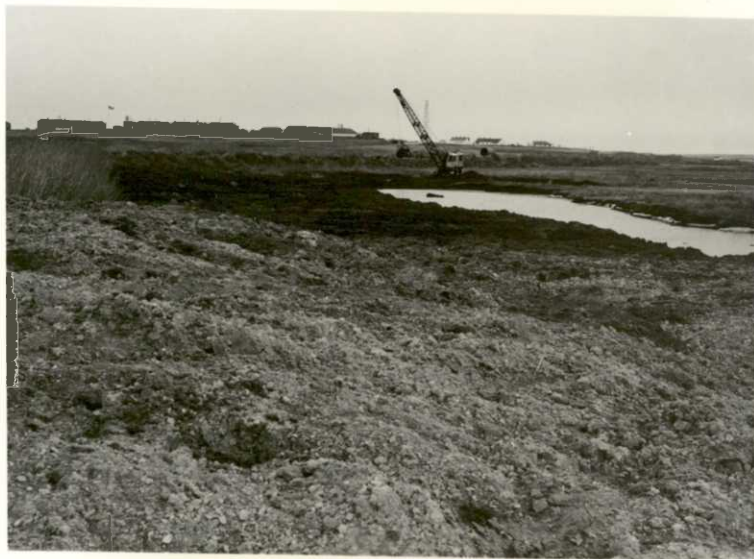
Dragline making a fill on Dike No. 3.
