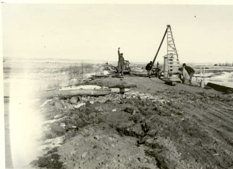
Making a fill on County road west of Refuge and preparing to drive piling to raise County road bridge.
