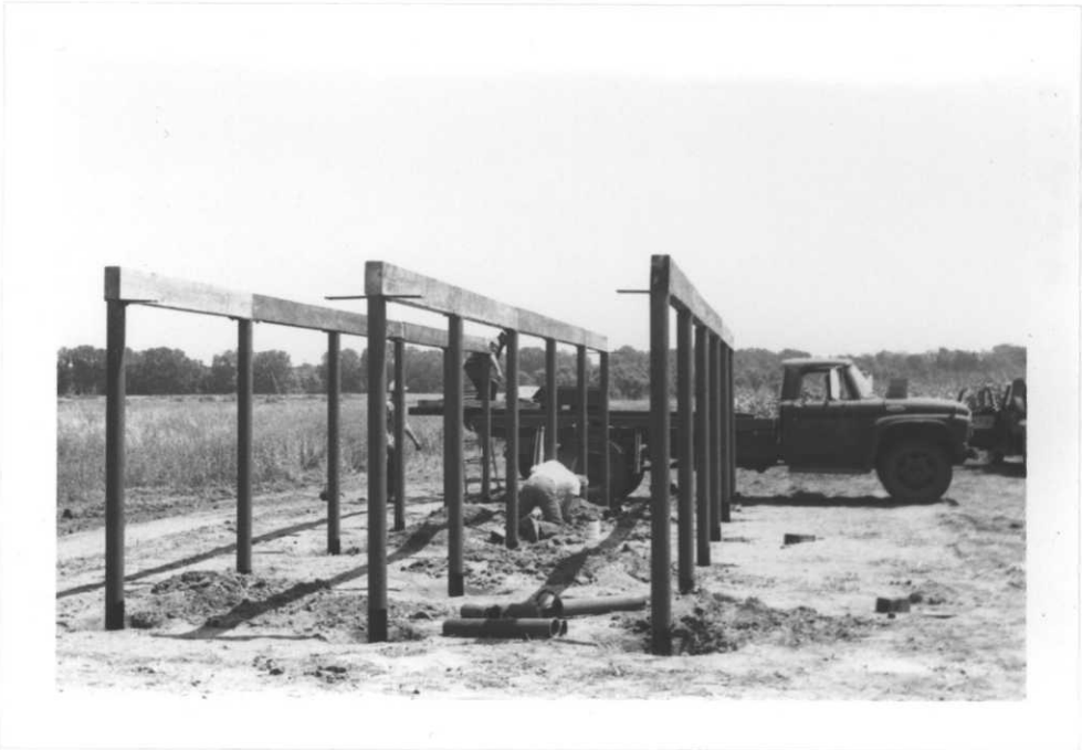
Refuge personnel constructed an observation stand at the south end of Fox Pond on Louisa Division.
