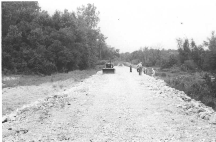
.....capped with 3-inch rock to provide a smoother driving surface.
