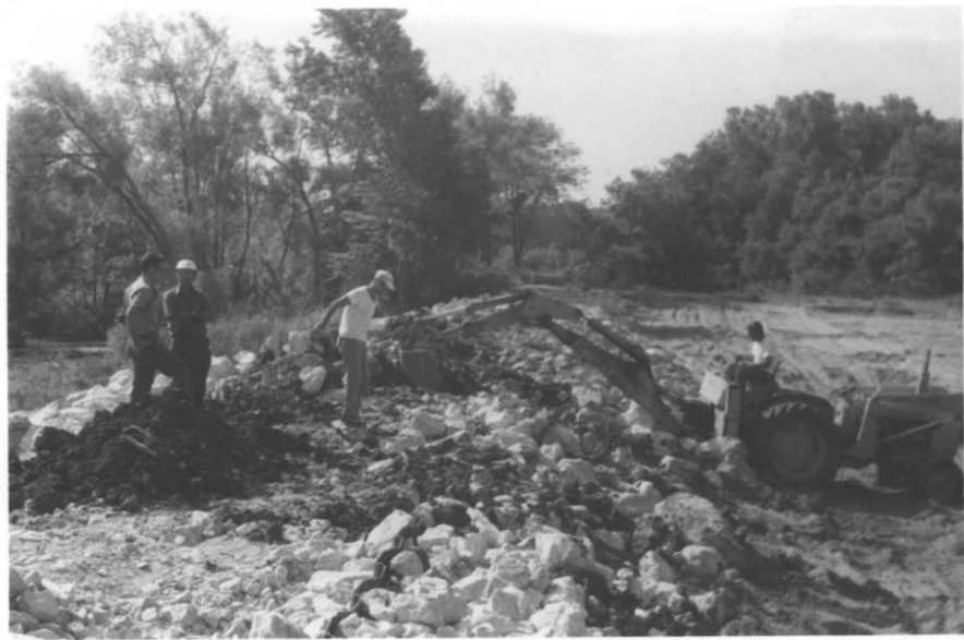
The structure was riprapped with 12-inch rock and...
