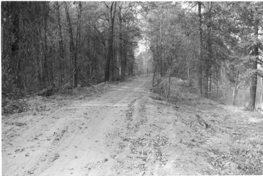
Roughed out section of road along Ditch 10
