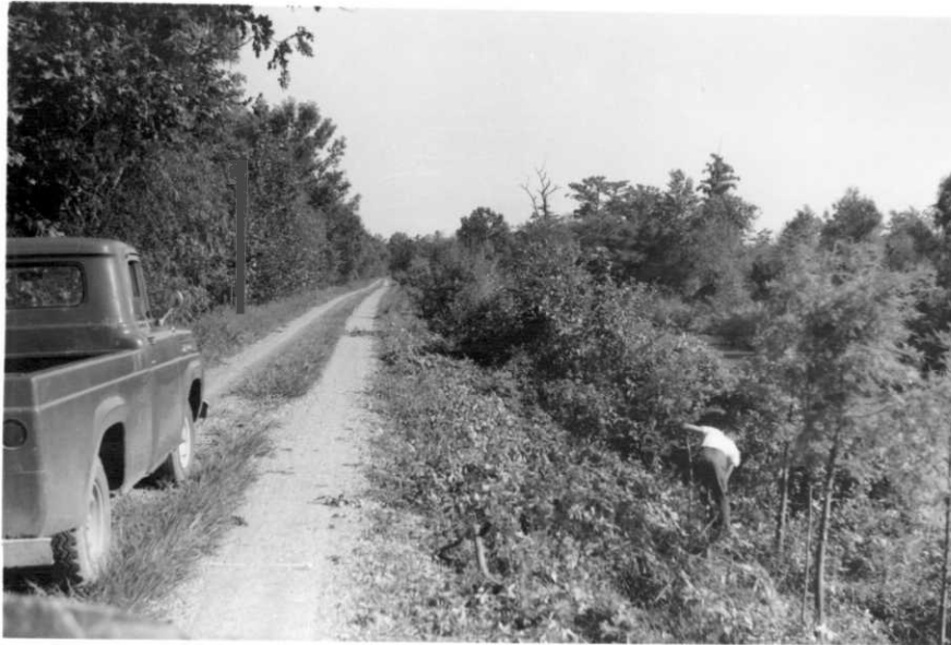
Start of cypress release clearing along Ditch 6
