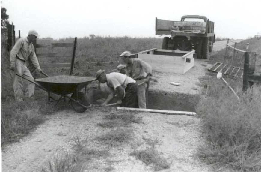
Cattle guards for G-3 and G-4 being constructed
