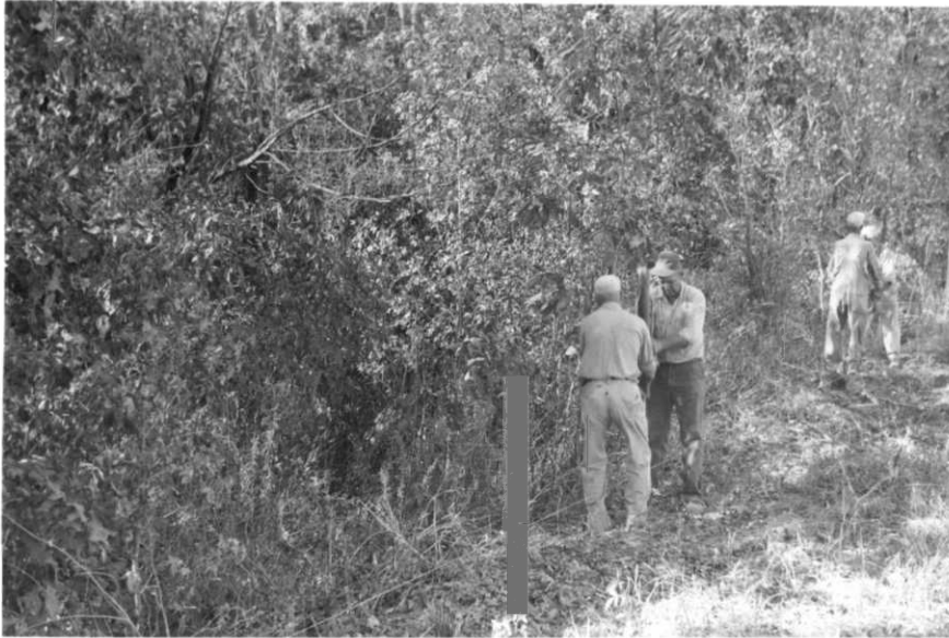
APW crew constructing north boundary fence
