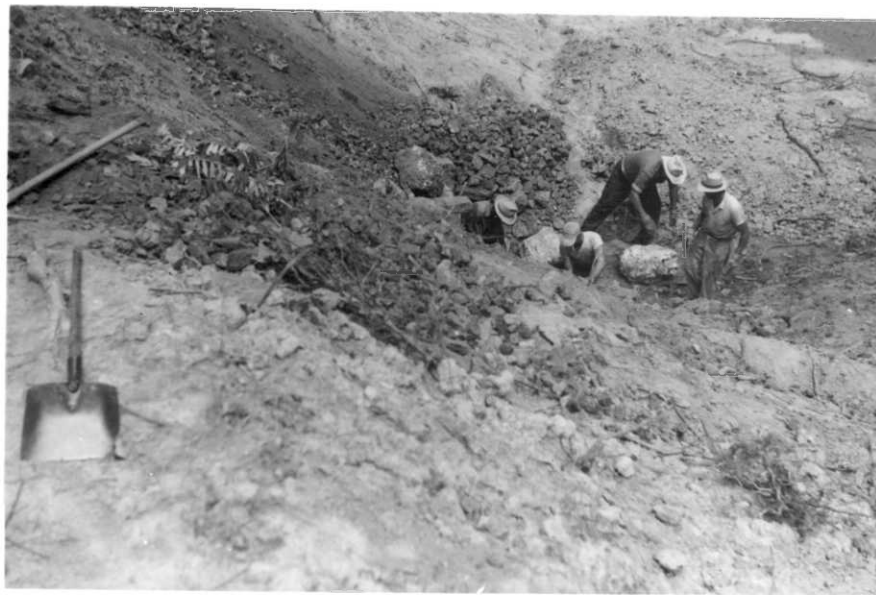
Rip-rapping of large earthen fill by APW crew
