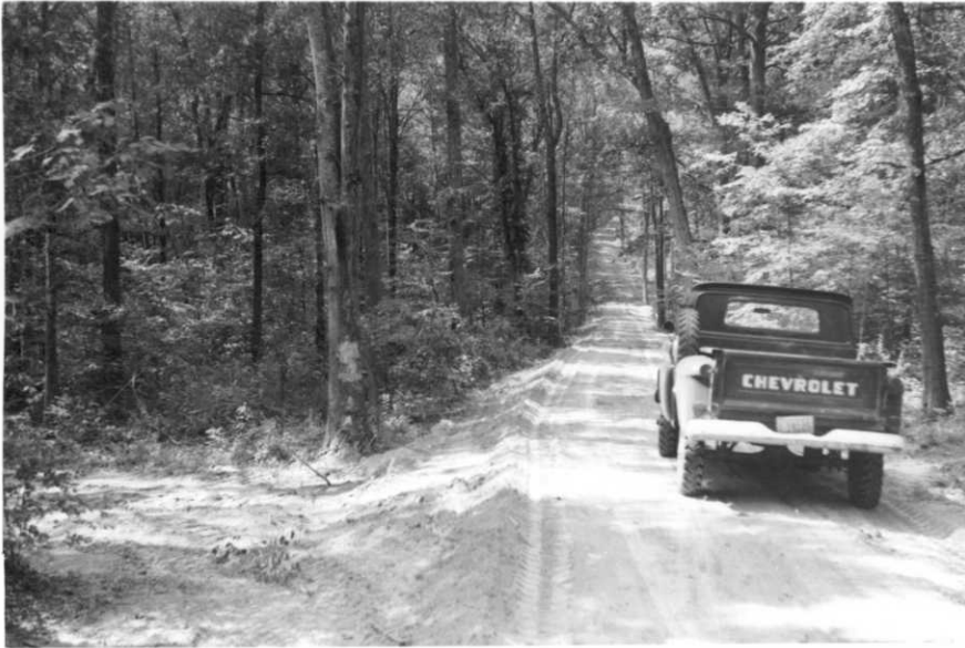
Completed section of westside fire & timber access trail
