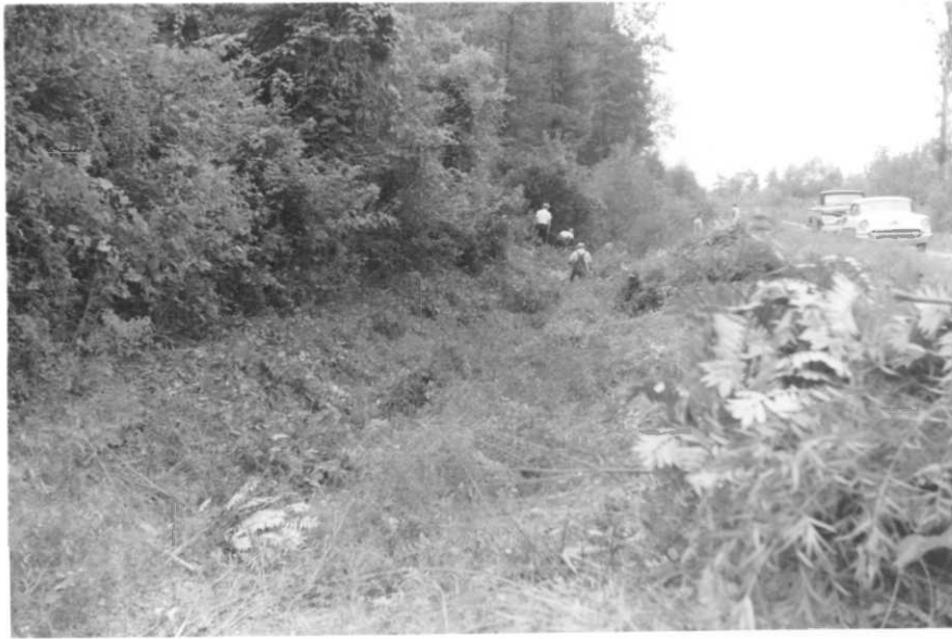
APW crew working on ditch clean-out
