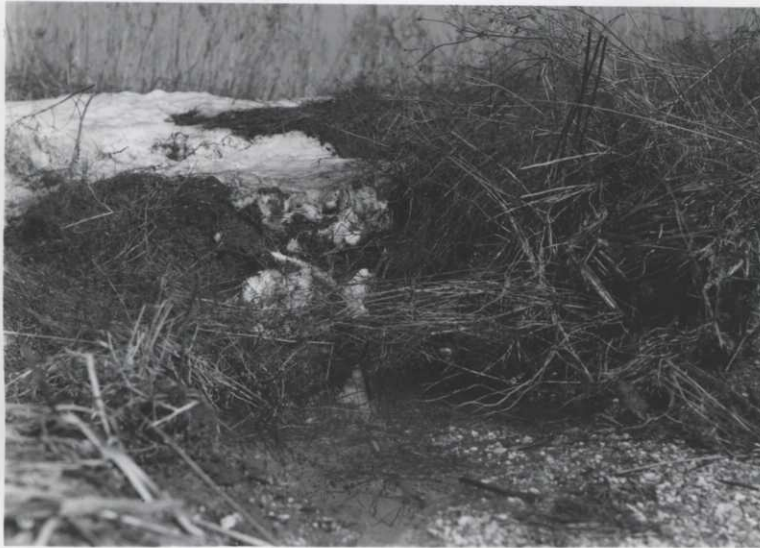
Washout through dam 341 caused by muskrats. R 142 - 4 - 5
