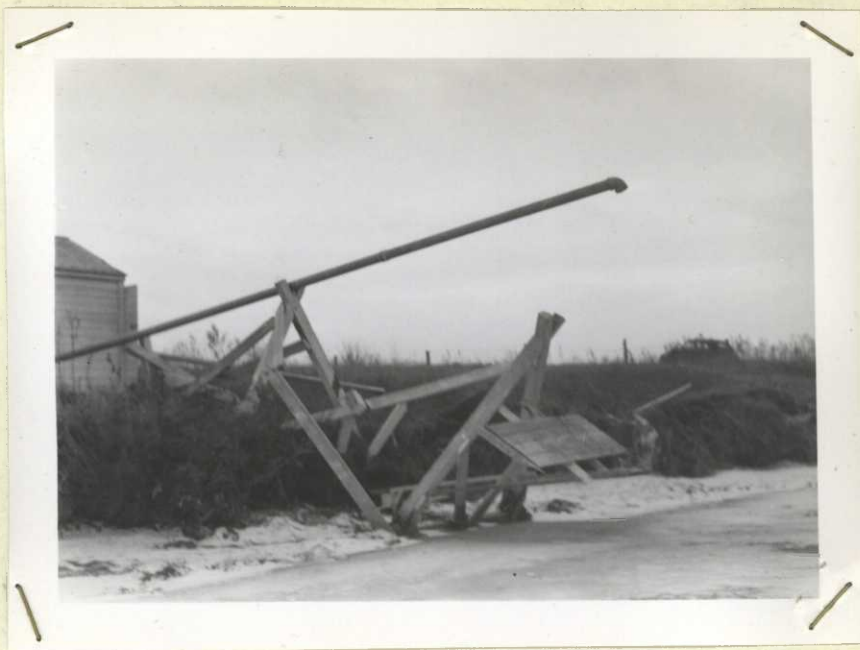
Damage by ice to nursery water pipes. R 142 - 3
