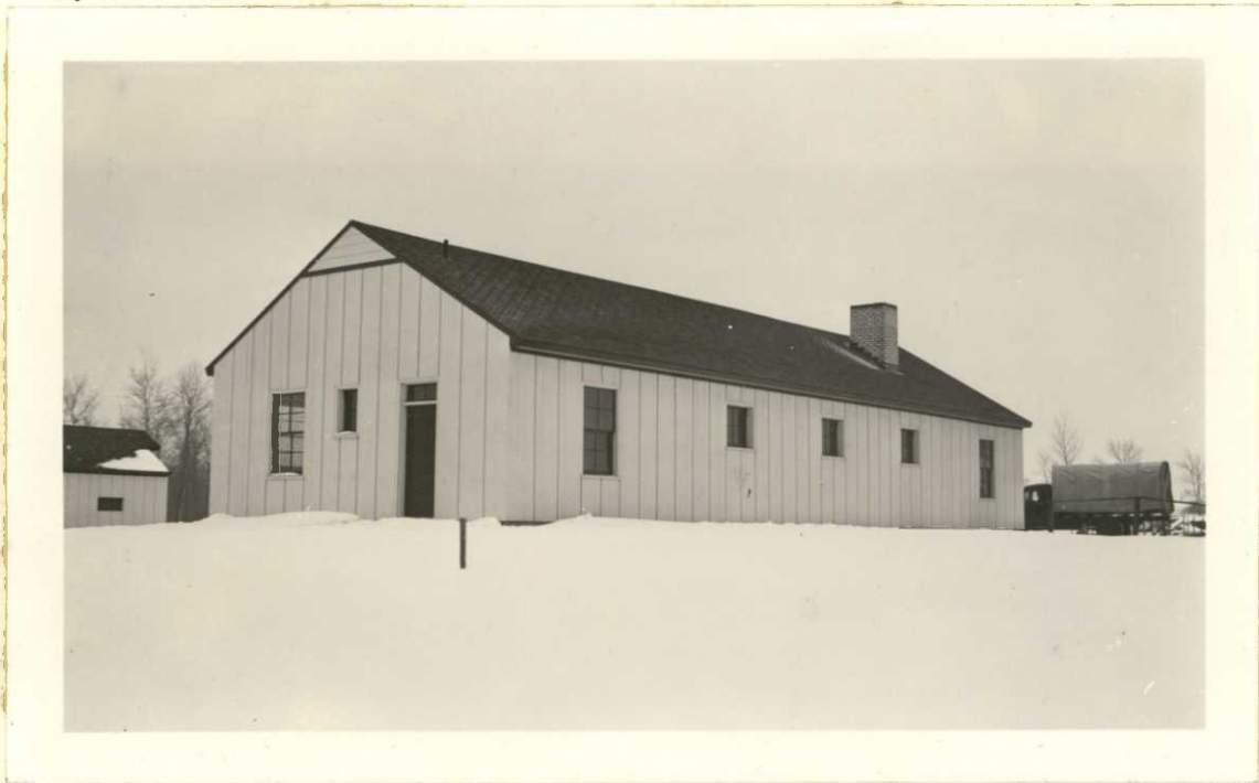
One story, frame, double board walls, composition-asphalt shingle roof, concrete floor thruout, concrete basement 13 x 25 where lighting system, furnace and water system are located, garage storage for three cars, work shop, office, laboratory, Hot water heat, electric lighted and shower bath, size: 26 x 72 x 9.
