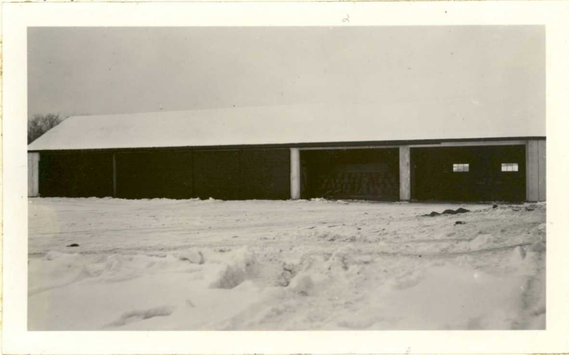
One story, frame, composition-asphalt shingle roof, concrete foundation, dirt floor, not heated nor electric lighted, size: 28 x 106 x 9.
