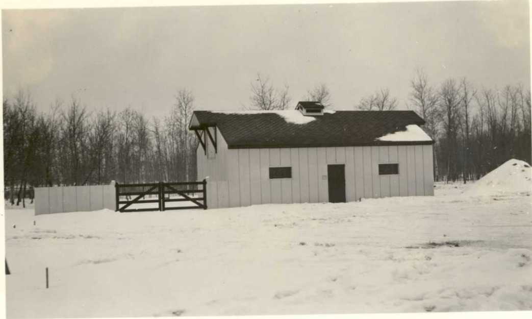
Frame, double board walls, composition-asphalt shingle roof, concrete floor, electric lighted, running water, size: 22 x 40 x 11.
