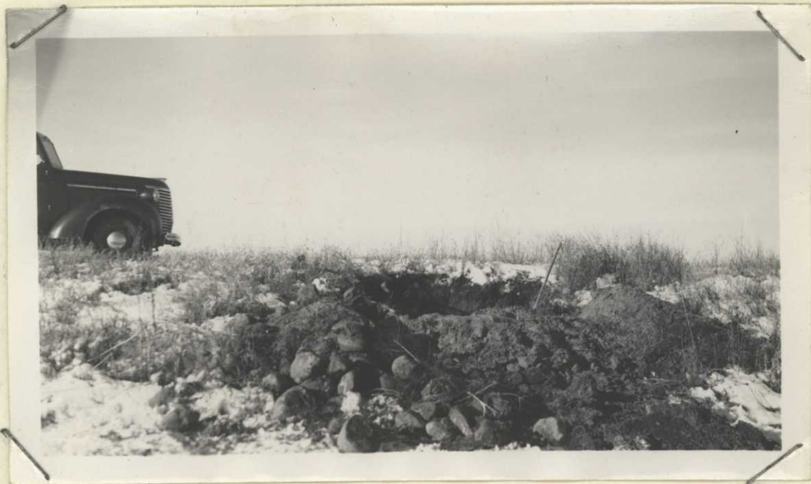
Chase Lake Easement Refuge; Dec. 14, 1944. View of Muskrat burrow dug out in dam. R-54-6.
