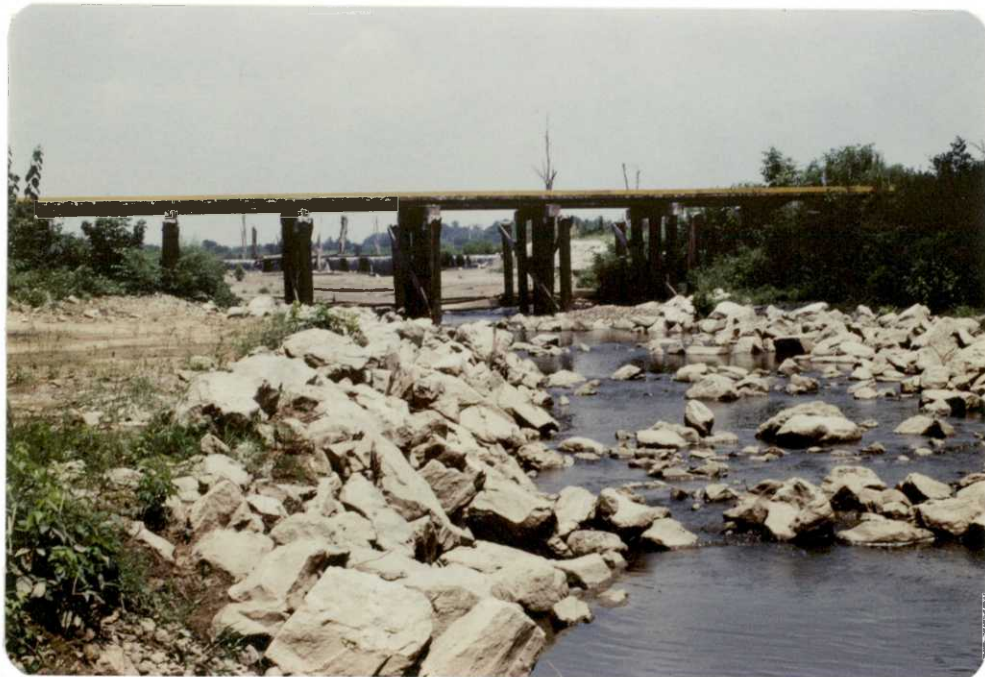
White bass spawning area below bridge at Little Creek impoundment. Large riprap to hold gravel from washing in the spring.
