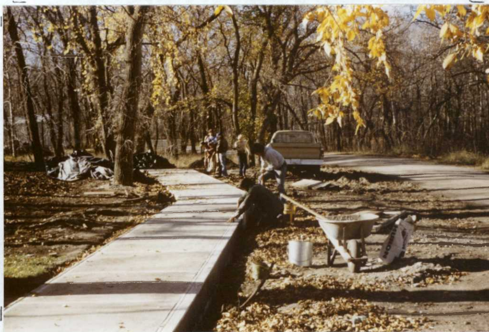
Figure 3. Constructing 200 feet of sidewalk from visitor's parking area to office building
