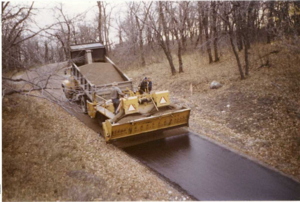
Figure 4. Applying seal coat to preserve roads.
