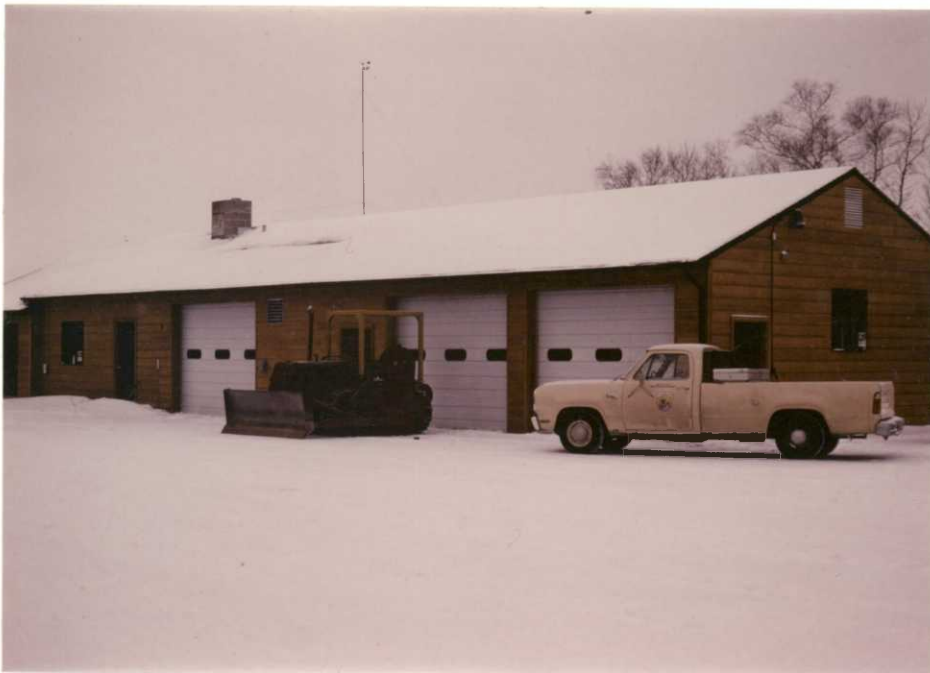
Post ARMMS rehab with insulated overhead doors, smaller triple glazed windows and 2" of foam insulation and siding over the concrete block. Birger November 1984
