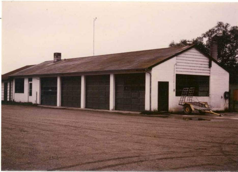
Refuge shop - Pre ARMMS rehab. Note the heavy wood overhead doors and large single glazed windows. Birger July 1984
