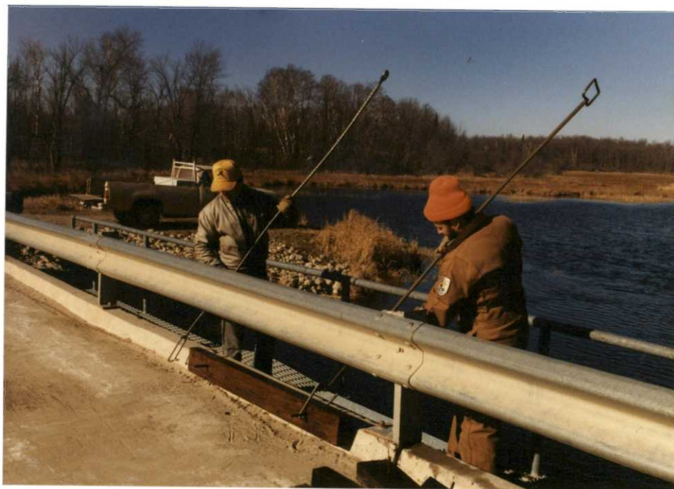
Installation of stoplogs at control structure.
