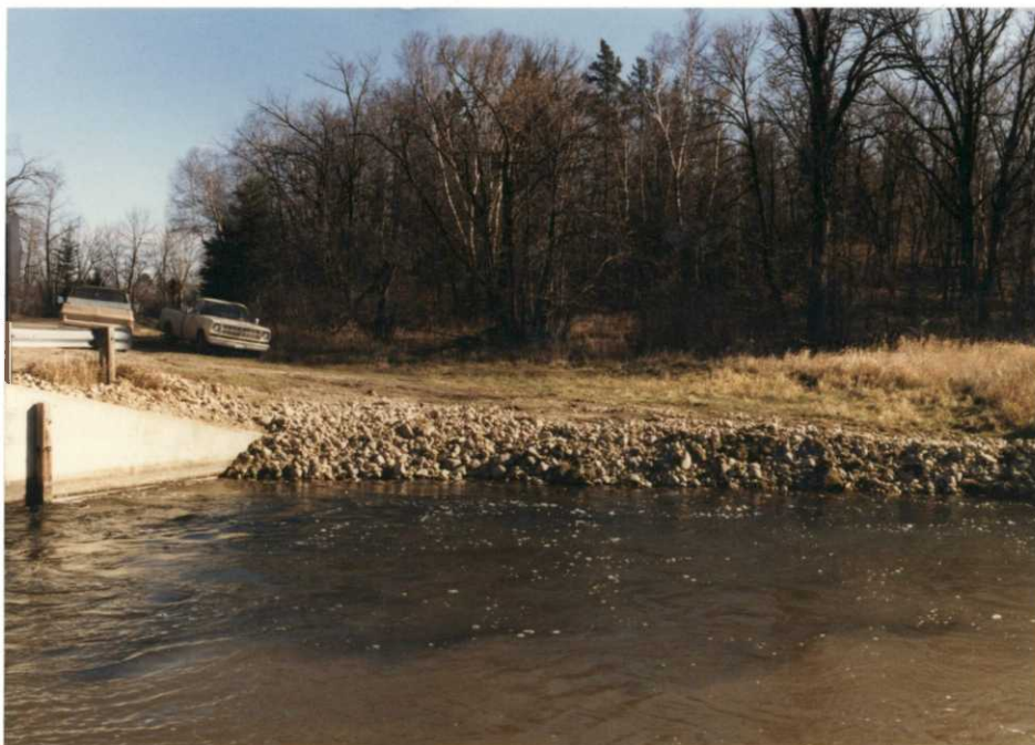
Riprap used to stablize shoreline downstream from Mitchell Dam. KMC 1985
