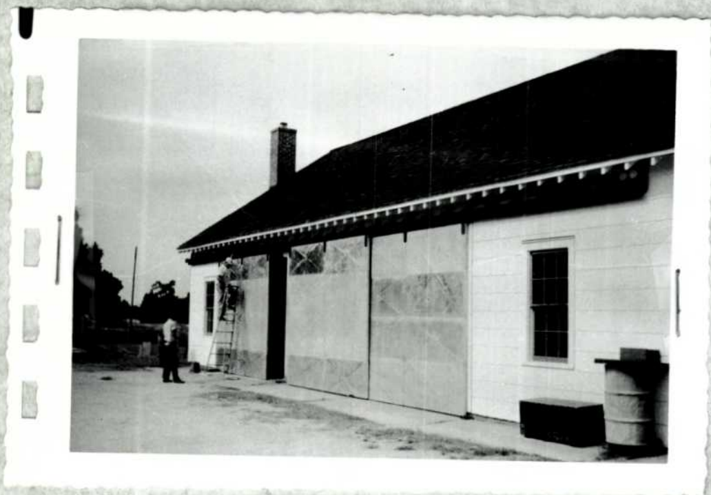
Swinging new, metal covered Service building doors
