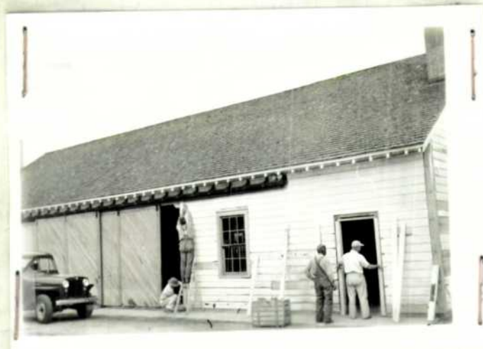
Preparing doors and windows of service building for covering entire building with asbestos-cement siding.
