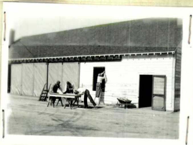
Preparing doors and windows of service building for covering entire building with asbestos-cement siding.
