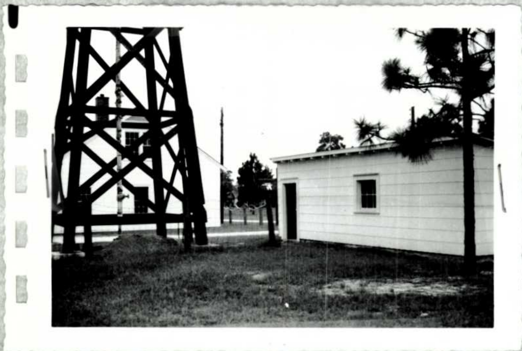
Pump house completed outside. To be insulated and sealed inside.
