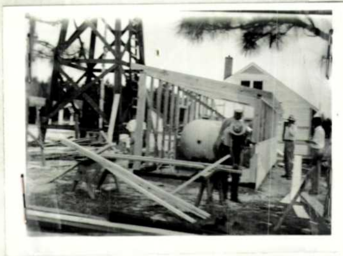
Pump House being constructed by refuge personnel.
